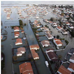
La Faute-sur-mer, western France after Xynthia storm, February 28 2010
