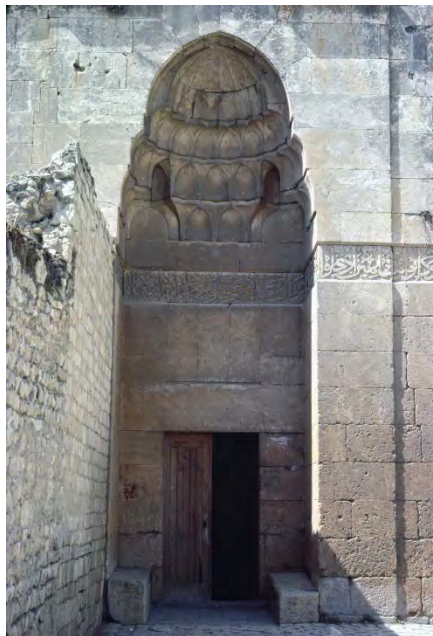
Figure 15 & 16. To the left is the muqarnas portal elevation and to the right is the view of view of muqarnas vault. Yasser Tabbaa Archive, 1990 developed, Aga Khan Documentation Center at MIT.
