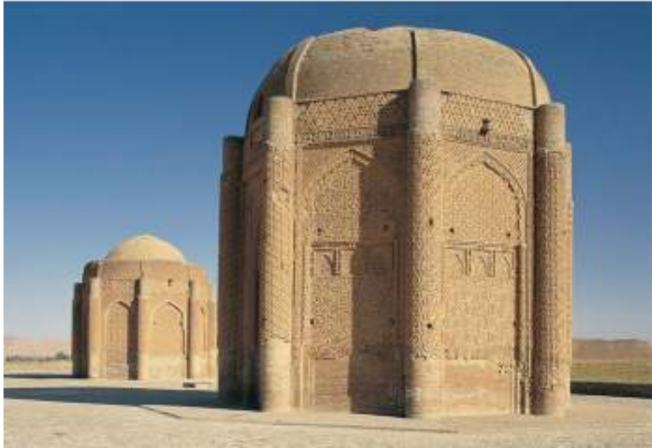
Figure 69. Kharraqān towers A.D.1067 and A.D.1093 Kharraqan region of northern Iran, near Qazvin
