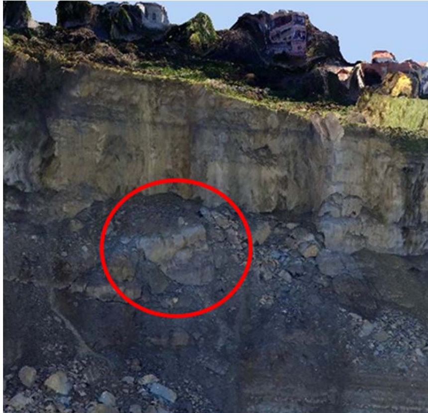
Figure 17: Wedge previously supporting the Blue Marl (Picture generated form Point cloud 3D representation)
