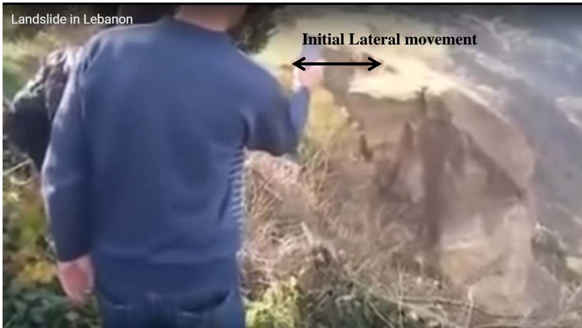
Figure 16: Snapshot from video of landslide showing a lateral displacement of the rock mass with a gap created between it and the stable ground
