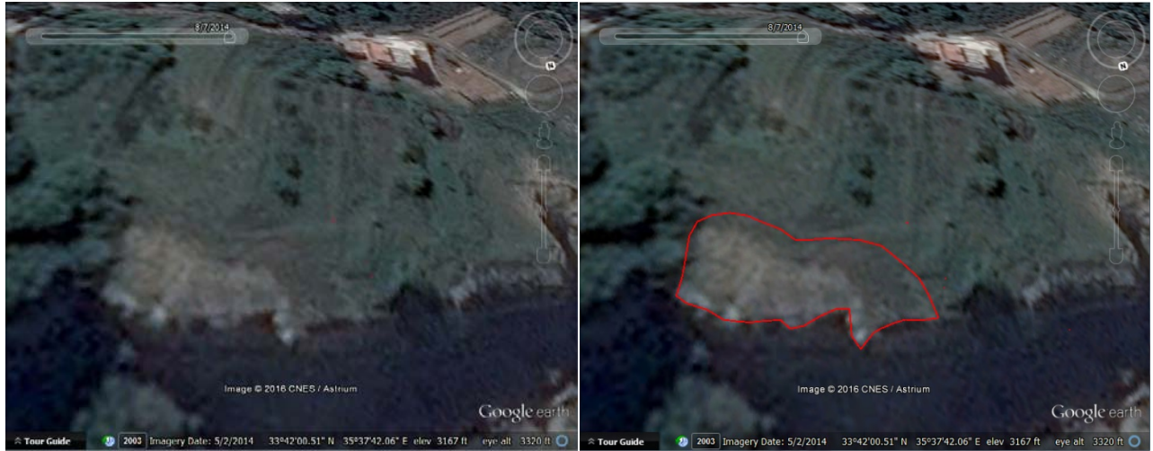
Figure 15: Change in color of grass as joints open and cut water supply prior to failing in August 2014- Red line presents 2015 failure zone (pictures from Google Earth Pro)
