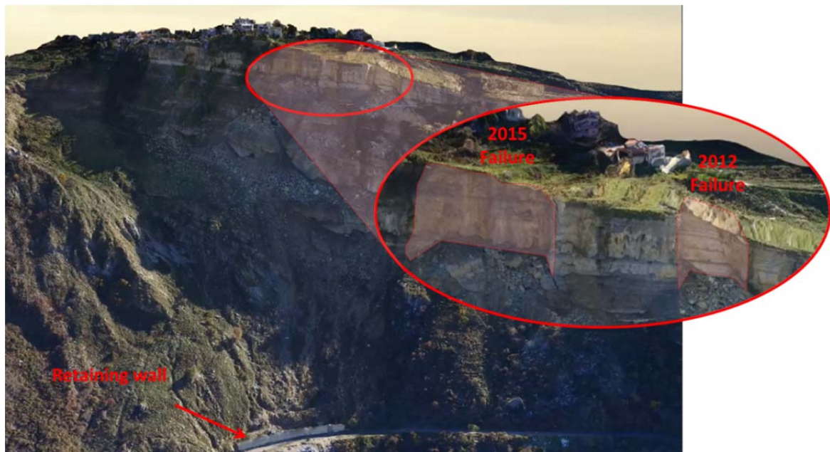
Figure 3: Location of the 2012 and 2015 landslides (Picture generated form Point cloud 3D representation)
