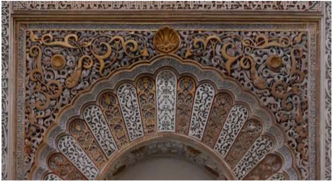
Figure 15 Mihrab detail – voussoirs and spandrels
