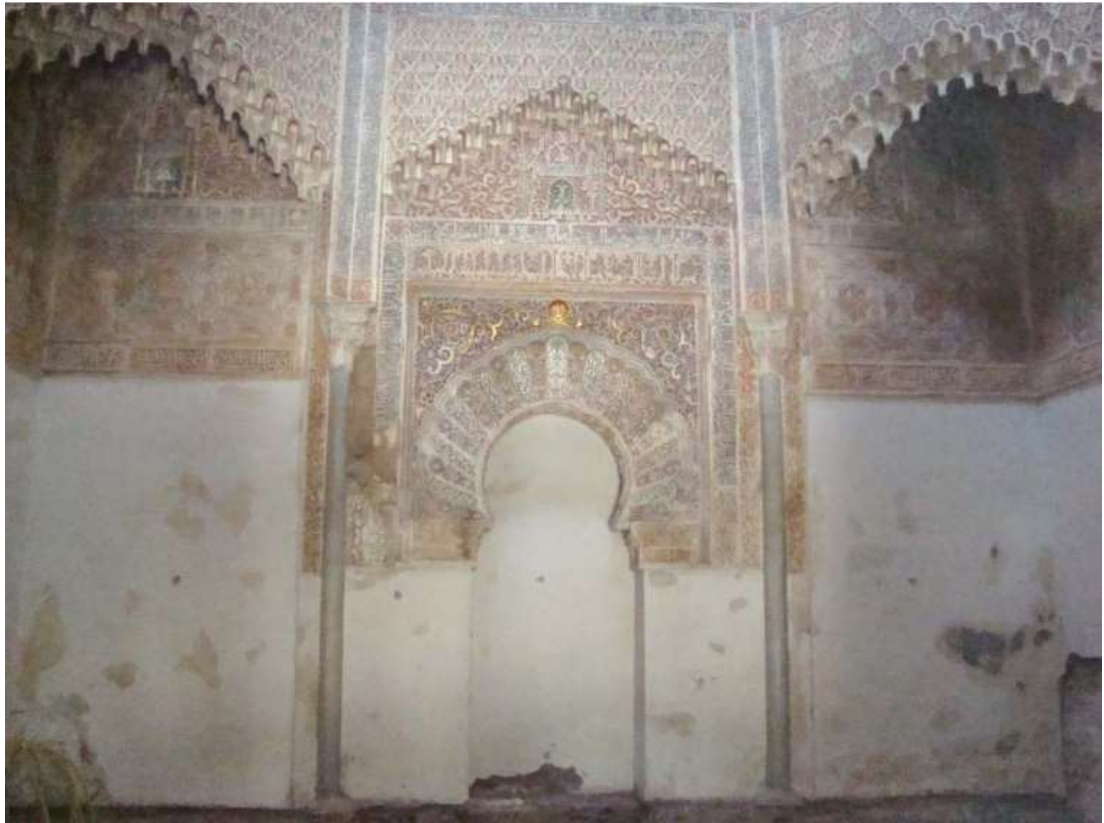
Figure 9 Mihrab niche before the intervention
