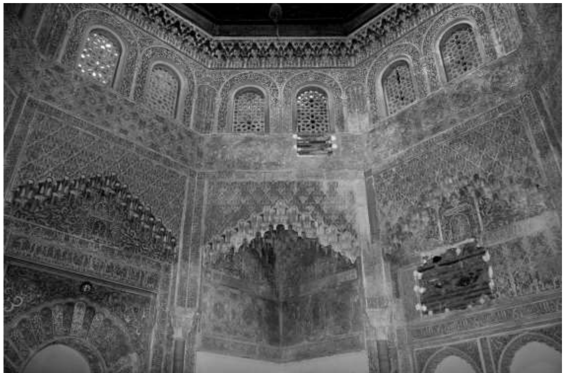
Figure 10 Prayer hall – State of the plasterwork before the restoration
