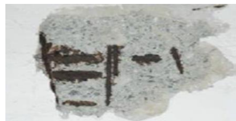
Figure 4: Reinforced ceiling concrete deterioration (Mydin et al., 2017).
