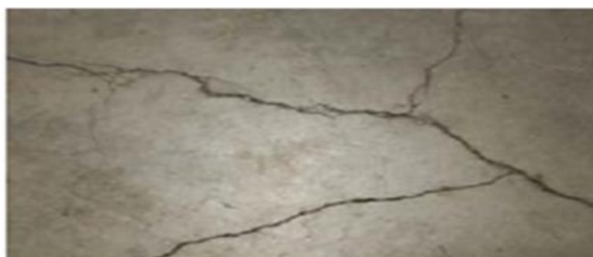
Figure 3: Major horizontal and vertical cracks on a concrete base foundation (Mydin et al., 2017).
