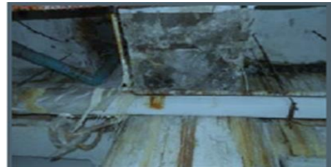
Figure 2: Razed paint structure and heavy equipment corrosion in mechanical rooms (Mydin et al., 2017).
