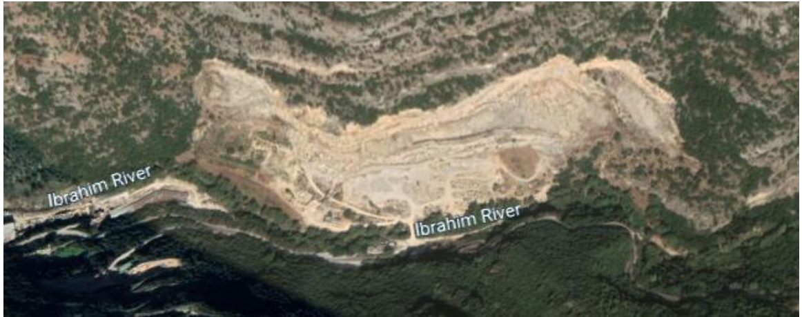
Figure 18: Google Earth image of the quarried slope detected in Halate, Jbeil
